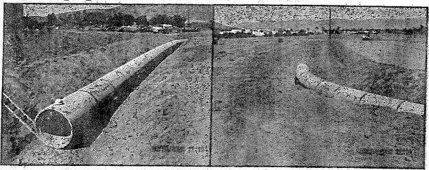
The 48" concrete storm drain is being placed along old Pico Street from West to East. This storm drain will direct offsite sheet flow from the East.
