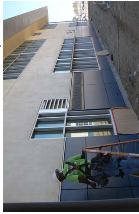
August 2011—Phenolic panels being attached to exterior base of both buildings
