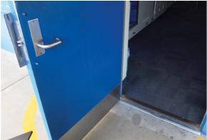
Door hardware and threshold visually appears to comply with barrier-free requirements.
