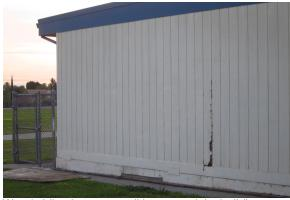
Wood siding in poor condition at modular building.
