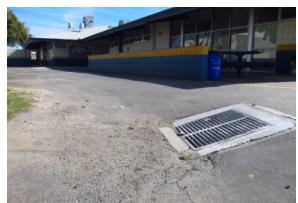
Significant slope issues at AC paving and walkways across campus.
