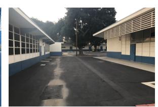
Evidence of ponding water at asphalt paving.
