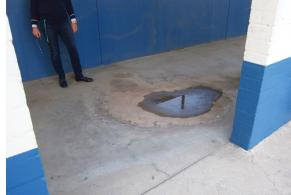
Ponding water at concrete paving.
