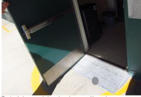
Typical door and door hardware, with no-longercompliant ramped threshold.
