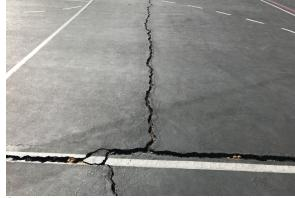
Significant cracking, typical across asphalt paving.
