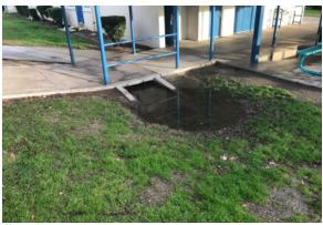
Flooding on planting area at clogged drain.
