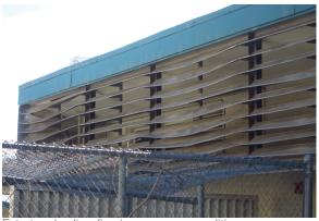
Exterior shading fins in very poor condition.
