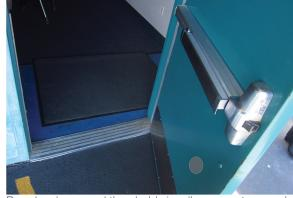
Door hardware and threshold visually appear to comply with barrier-free requirements.
