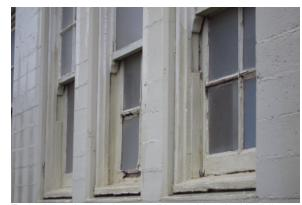
Typical exterior window condition at historical building, highly deteriorated.
