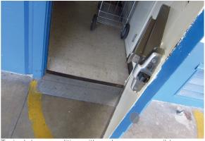
Typical door condition with no-longer-accessible ramped threshold.
