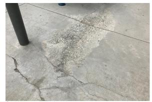
Cracking and weather damage at concrete paving.
