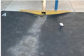
Evidence of ponding water at asphalt.
