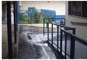
Significant grading and ponding issues at asphalt, especially around portable classrooms.
