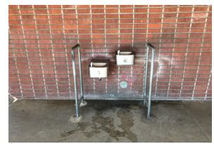
Significant effluorescence on brick walls at drinking fountains and other locations exposed to moisture.
