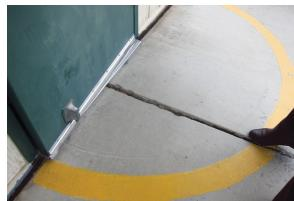
Significant separation at pavement joints.
