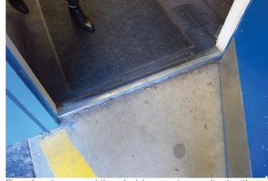
Door hardware and threshold are not compliant with accessibility requirements.
