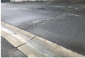
Wear and unevenness at asphalt paving.
