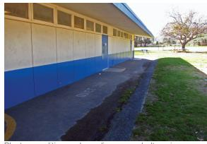
Plaster condition and ponding on asphalt paving.
