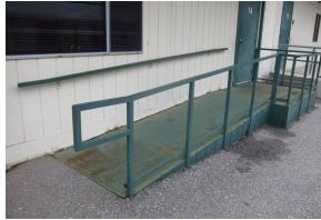
Rusted ramps and evidence of ponding water at portable buildings.
