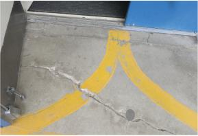
Door threshold and cracking at concrete at door landing.
