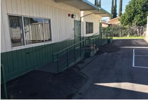
Inaccessible cross slopes at portable classroom building grading.
